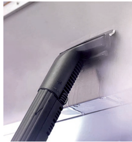
Steam exhaust cleaning
