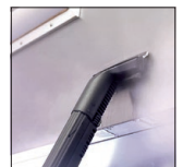
Steam exhaust cleaning
